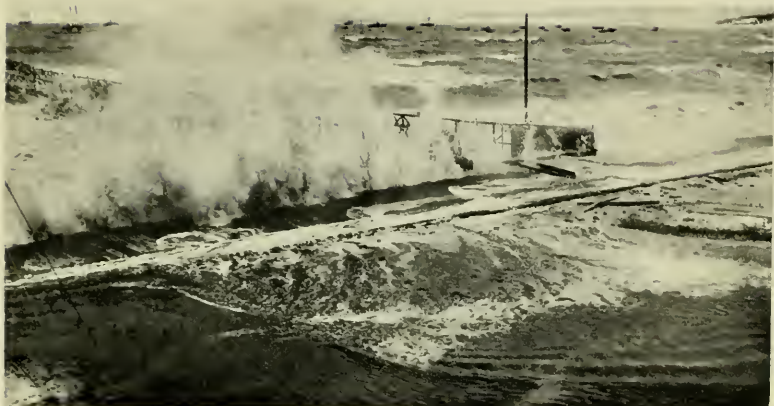
THE ROADS OF PUNTA ARENAS, SOUTH-WESTER BLOWING.
